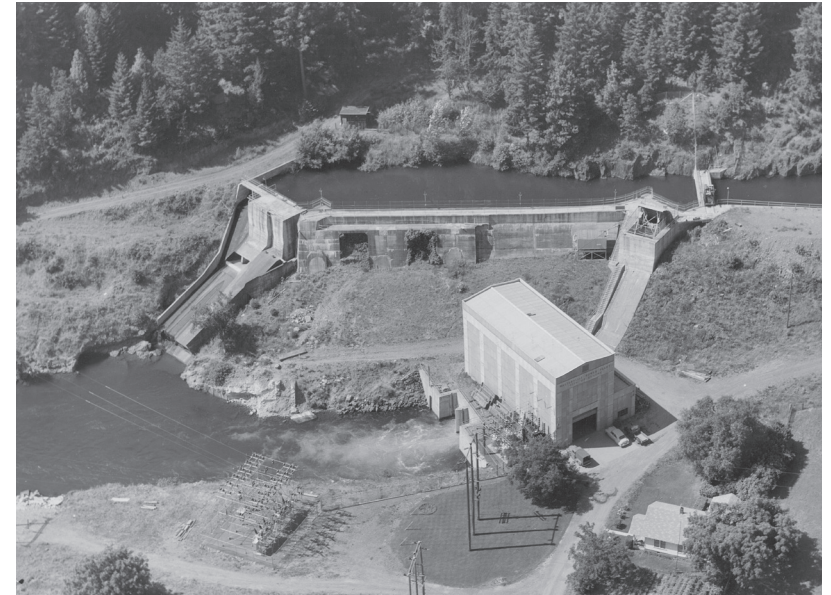
Walterville Canal Forebay and Powerhouse, 1940
