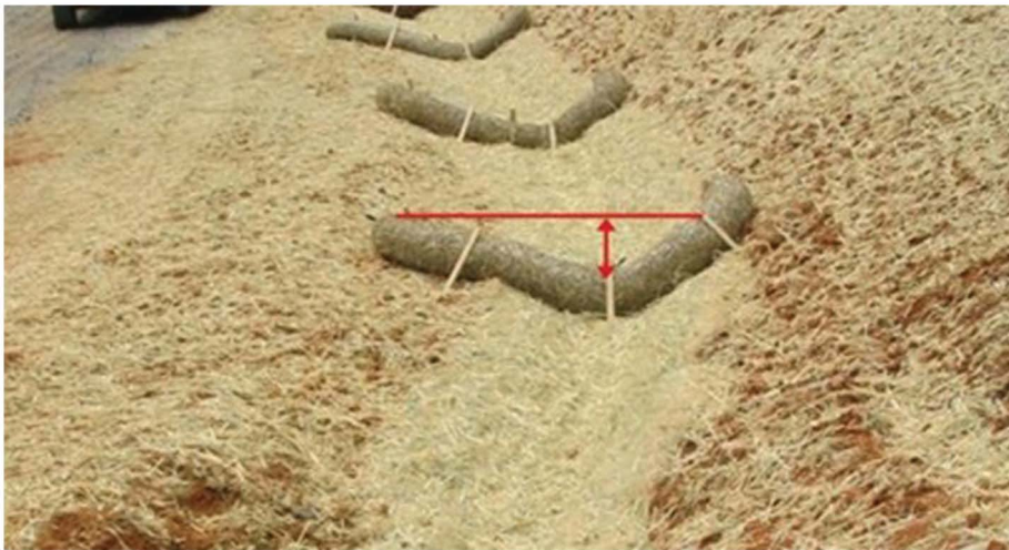
Photo 1: Check Dam placement in drainage swale
