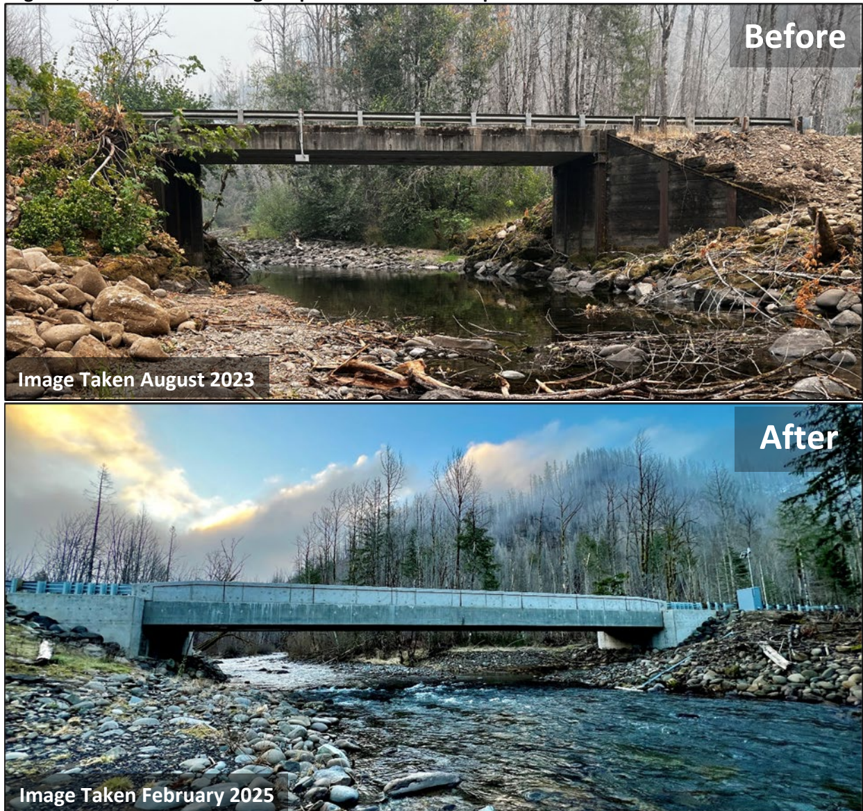
Figure 1-2: Quartz Creek Bridge Replacement Work Completed in 2024
